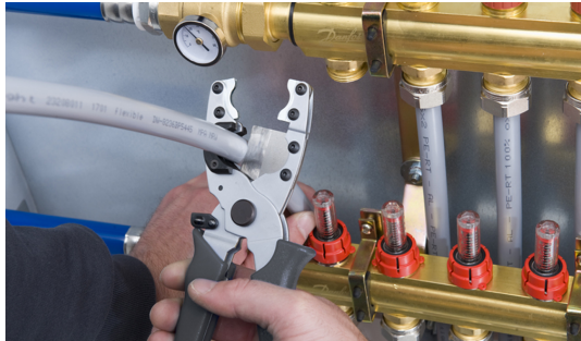
Fig. 1: Before connecting the heating circuit to manifold cleanly cut off FH composite pipe in the correct length.
