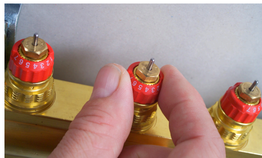
Fig. 8: Preset manifold valve for each heating circuit according to calculations and manifold data sheet.
