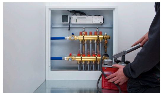
Fig. 6: Label the individual heating circuits. Carry out pressure test in accordance with the pressure test protocol.
