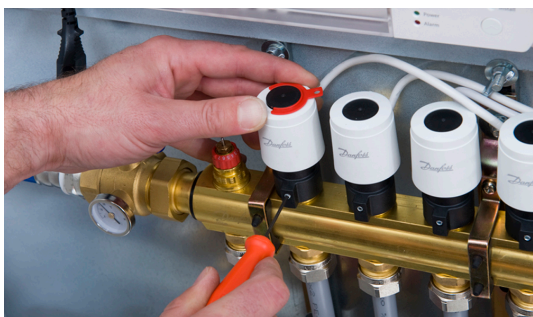
Fig. 9: Fix actuator to valve with a 2 mm Allen key and connect actuator and room thermostats via wiring centre or master controller.
